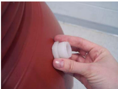
Putting in a threaded adaptor.
