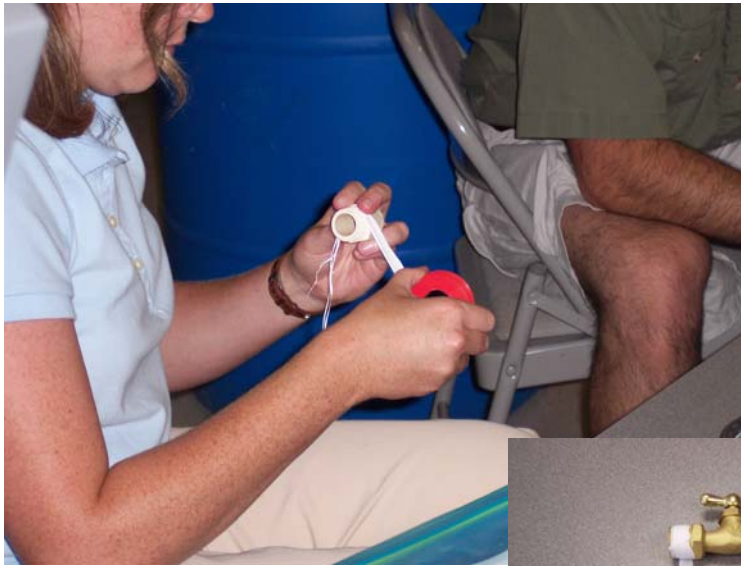
Wrapping tape around the hose spigot
